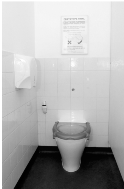
Figure 2. ULFT installed during the trials at WRc. (Photo courtesy of Phoenix Product Development)
